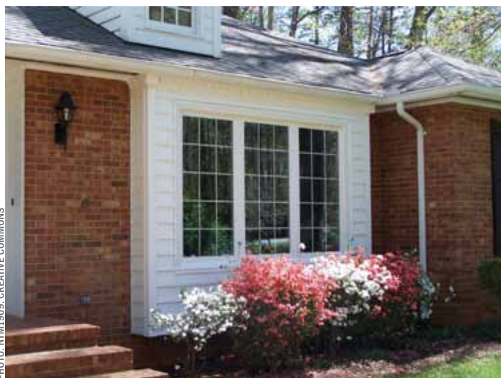
Installer's friend: Bushes and windows provide a great way to minimize the appearance of siding seams.
