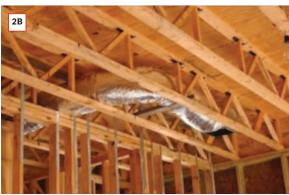
Avoid taking up slack with sharp bends [2A], which severely reduce airflow. Plan the framing package to include chases or trusses to accommodate ductwork [2B]. Ducts that are not stretched tight or that contain sharp bends can increase the equivalent length of the duct run by several multiples (see illustrations at left).
