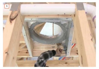
All ducts, whether rigid or flexible, should be sealed with UL-181-rated duct mastic. Duct tape has many uses, but sealing ducts isn't one of them.
