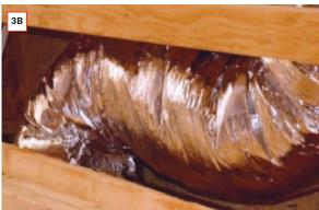
Lack of coordination among subtrades can result in bends and kinks to avoid piping, wiring, and framing components [3A]. To prevent the need for costly troubleshooting behind finished walls and ceilings, carefully inspect before drywall is installed to make sure there are no sharp bends or any kinks concealed behind framing [3B].
